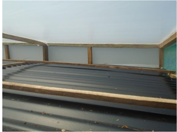
Figure 34: Piece of wood added to protect the plastic sheet when the trays are introduced
