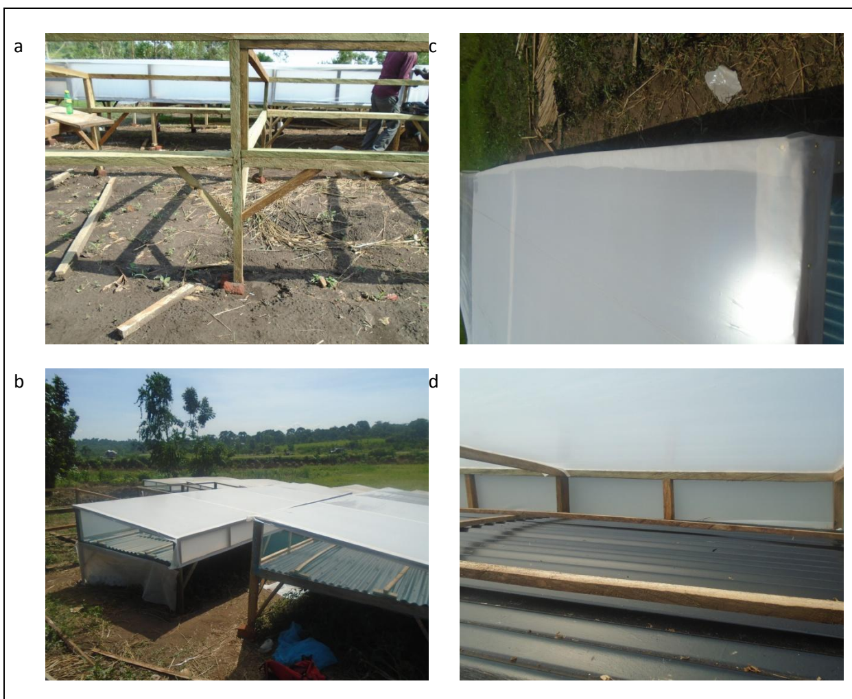
Figure 23: Improvements on the solar dryer. (a) Bricks insertion under the feet & added square on the side. (b) Plastic foil to close the dryer during the night. (c) Double layer of plastic foil. (d) Piece of wood introduced on the opposite side of the doors
