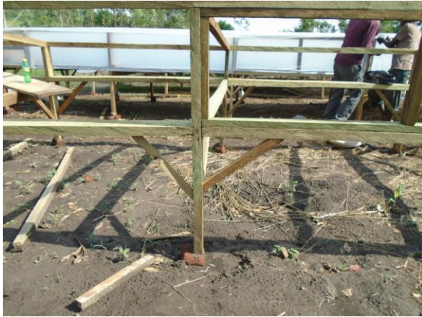
Figure 33: Squares added to improve the robustness
