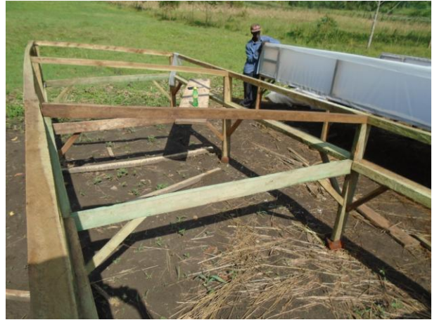
Figure 31: Picture of the ventilated solar tunnel dryer structure
