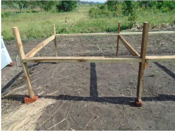
Figure 30: Picture of the ventilated solar tunnel dryer structure
